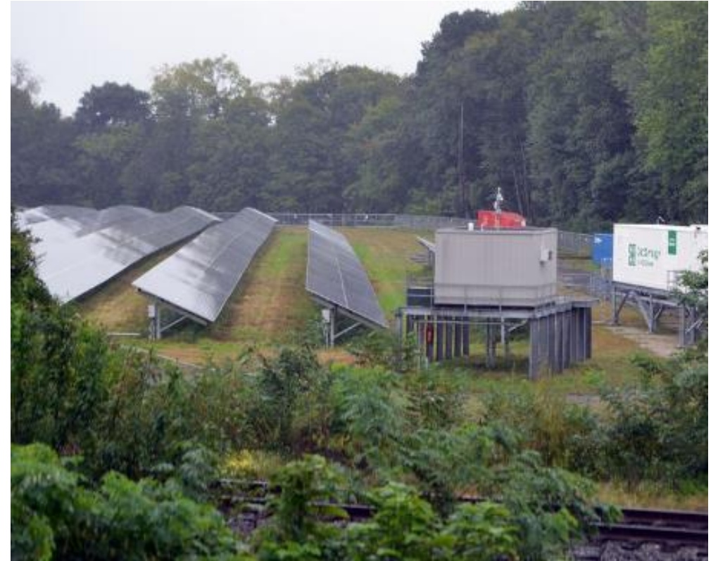
ENGIE North America and Holyoke Gas & Electric: The largest energy storage system (with solar) in Massachusetts, located at the site of the old Mt. Tom power plant.
